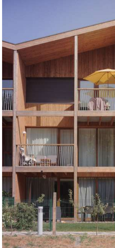
Structure bois - Tank, Nantes
