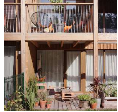
Structure bois - Tank, Nantes
