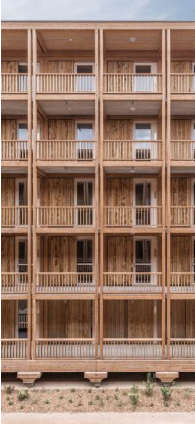
Structure bois - acau architecture, Genève
