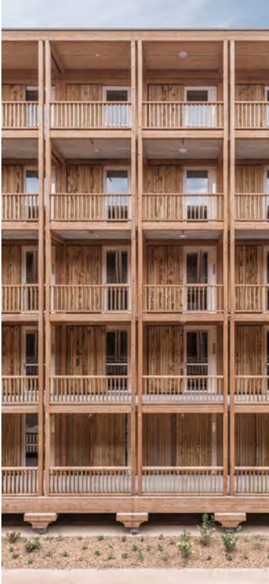
Structure bois - acau architecture, Genève
