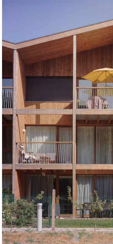
Structure bois - Tank, Nantes
