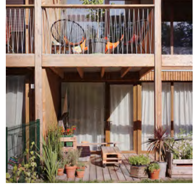
Structure bois - Tank, Nantes
